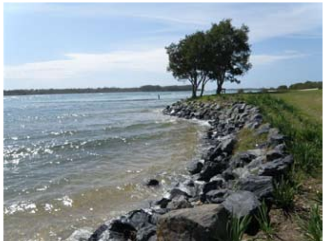
Plate 18. River bank stabilisation
