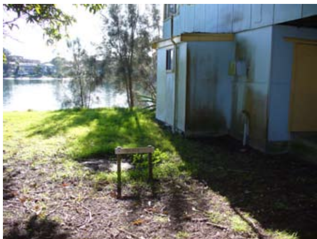
Plates 13 and 14. OSMS located close to the river
