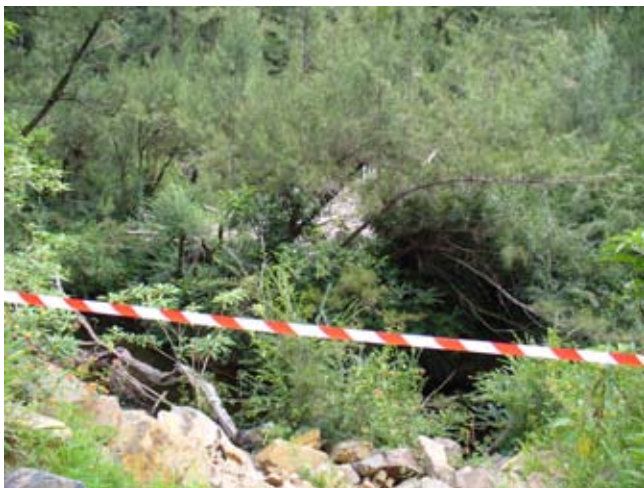
Plate 31. Kalang Road - Flood impact on rural roads and bridges
