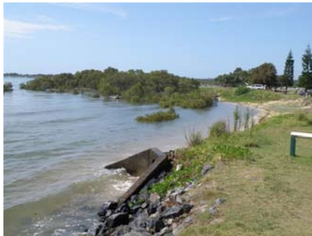
Plate 30. Stormwater runoff to river
