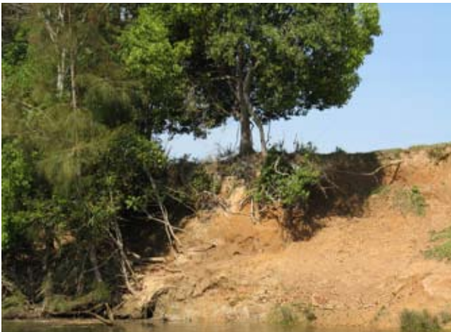
Plate 19. River bank erosion
