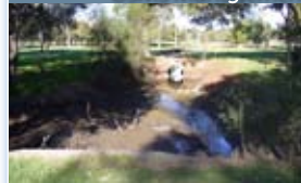
Stormwater & Construction Site Management
